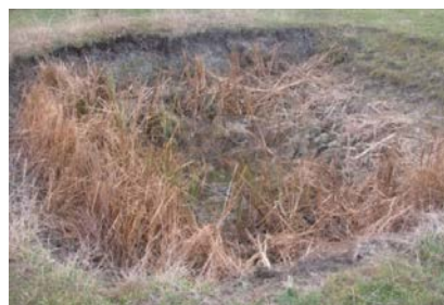
Fig. 2 – Silted soil profile with the presence of groundwater to the surface.
