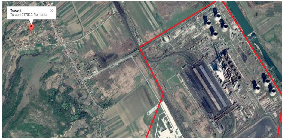
Fig. 1 – Monitoring area of Turceni Thermal Power Plant, Romania (Satellite map: http://satellite.worldmap.com ).
