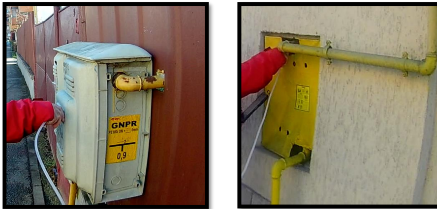
Fig. 2 – Example of the end-use points at which CH 4 concentration was estimated from the city center area and the residential area.
